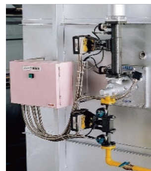
図4-1. IBS (Intelligent Burner System)
