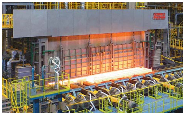
Walking beam type reheating furnace
