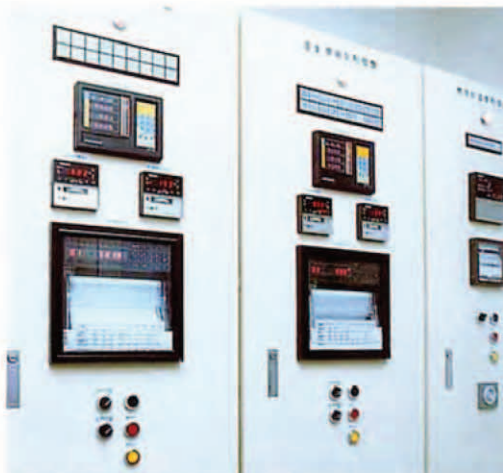
Temperature and atmosphere control panel incorporating a two-channel program controller
